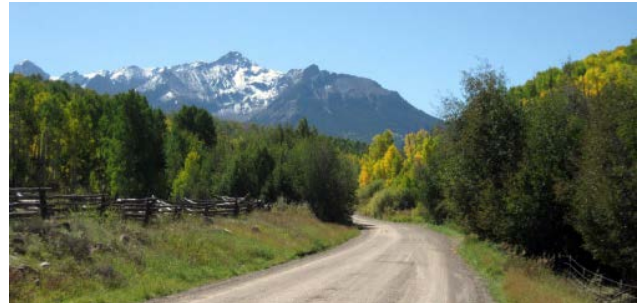
Example unpaved road owned by the U.S. Forest Service (Source: Unpaved Roads Less Traveled Blog).
