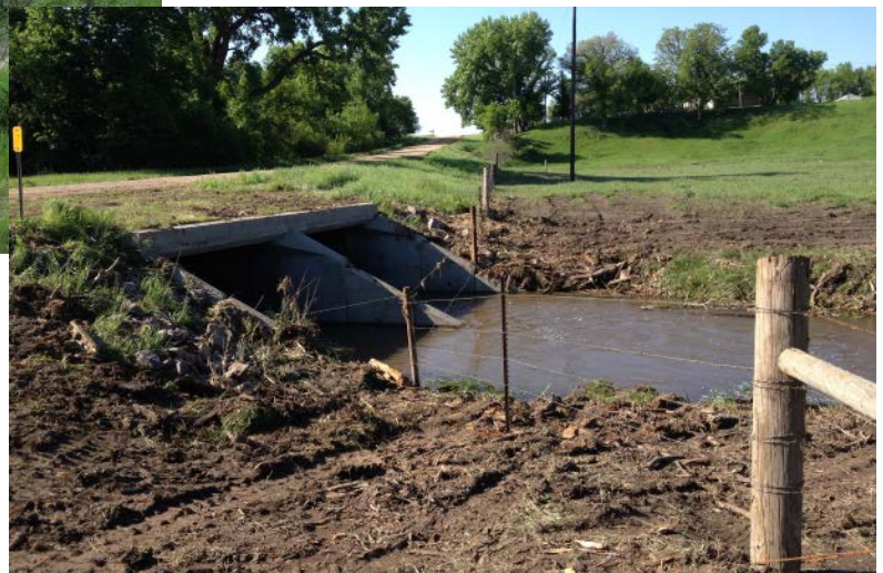
A large double box structure, completely plugged with debris after flooding and the same structure after debris removal and channel clean-up by a county maintenance crew.
